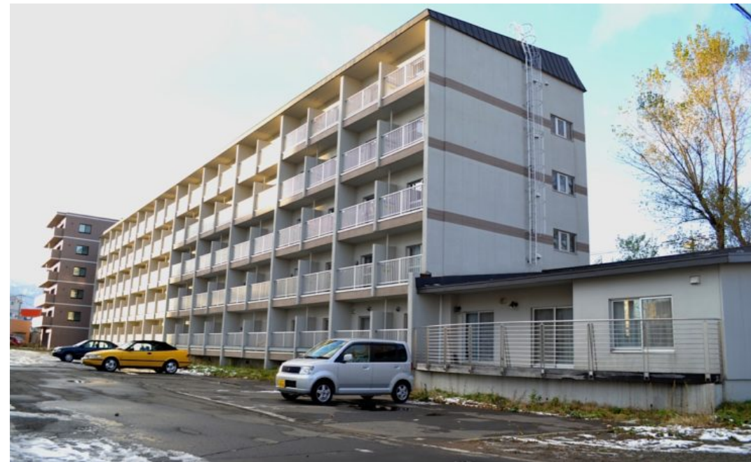
International House North 23 building 1
