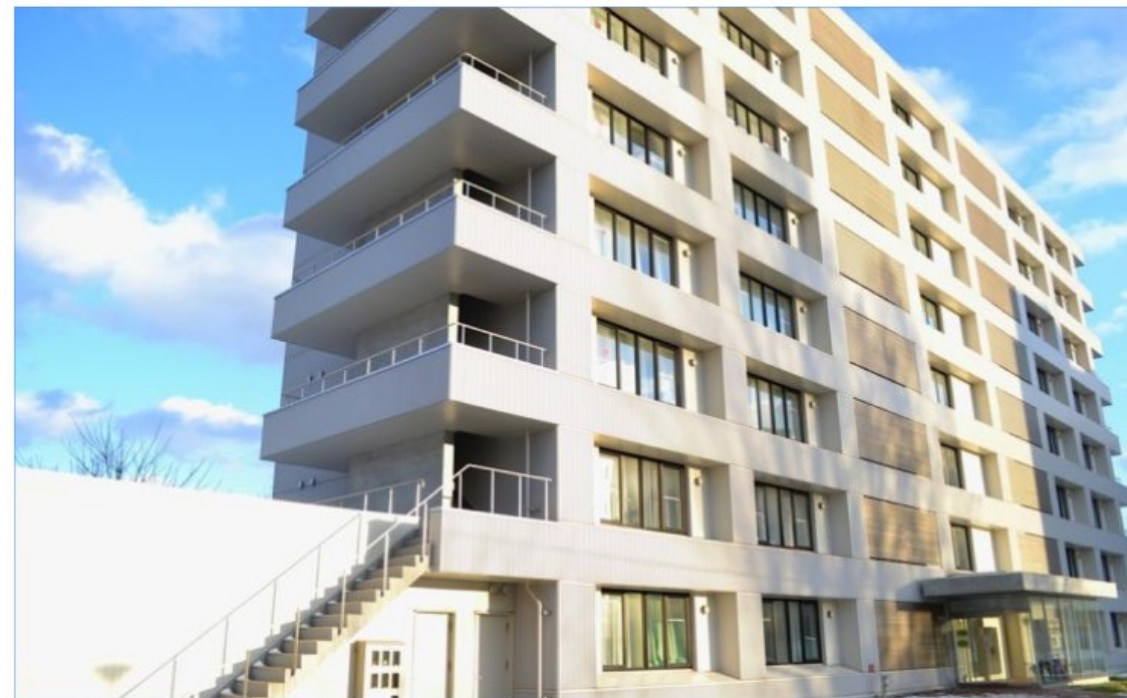
International House North 23 building 2
